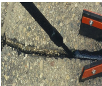
Crack Sealing
